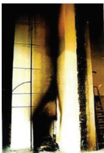
Figure 15: Damage of the test sample: render finishing
