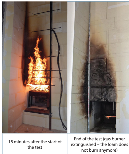
Figure 8: Fire of an ETICS without fire barriers during construction – Test according to DIN 4102-20 before rendering is applied (naked PIR product of class E)
