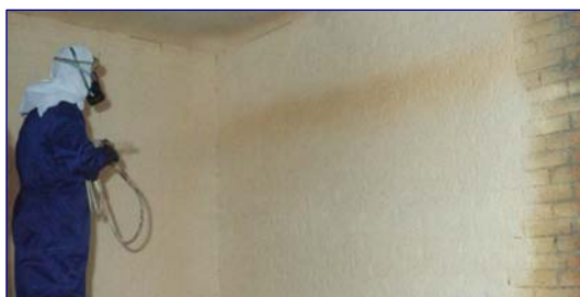
Picture 23: Spraying over a masonry wall
